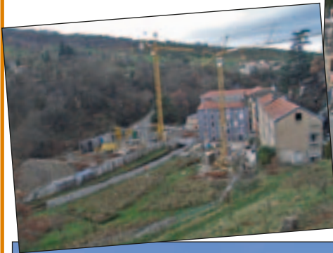
60. Renovation work. Notre Dame de l’Hermitage (2008).
